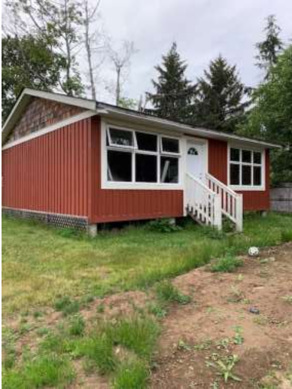
Figure 4: View of Main Access of Accessory Building (eastern side)
