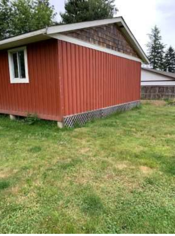
Figure 7: Southern (front-facing) Side of Accessory Building
