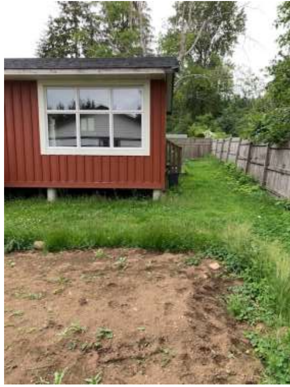
Figure 5: Accessory Building & Rear Lot Line (northern side)
