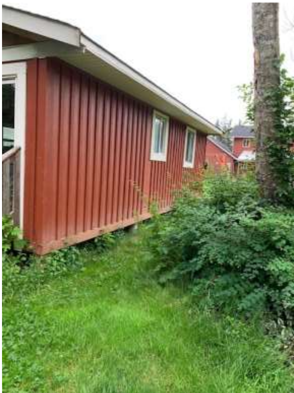
Figure 6: Accessory Building Looking Toward the House (western side)
