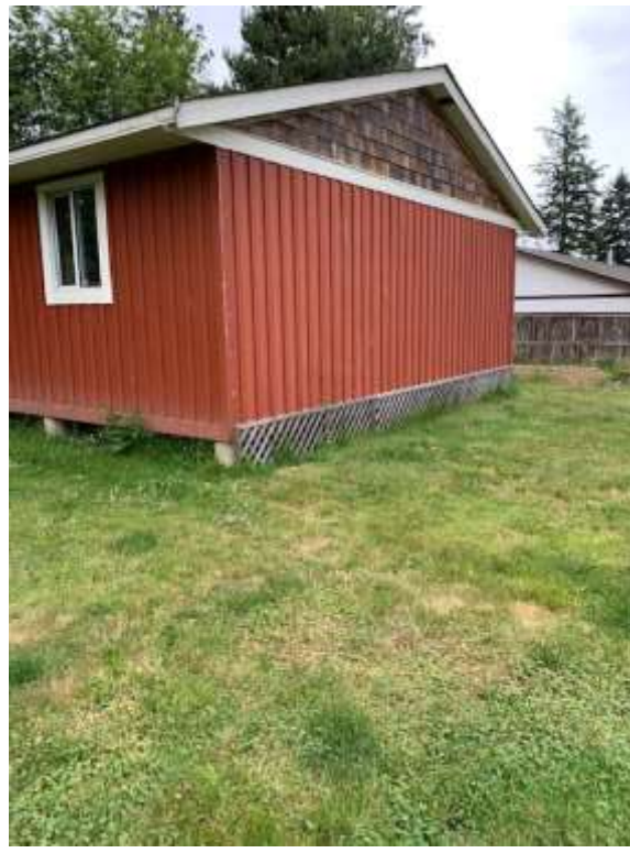
Figure 7: Southern (front-facing) Side of Accessory Building
