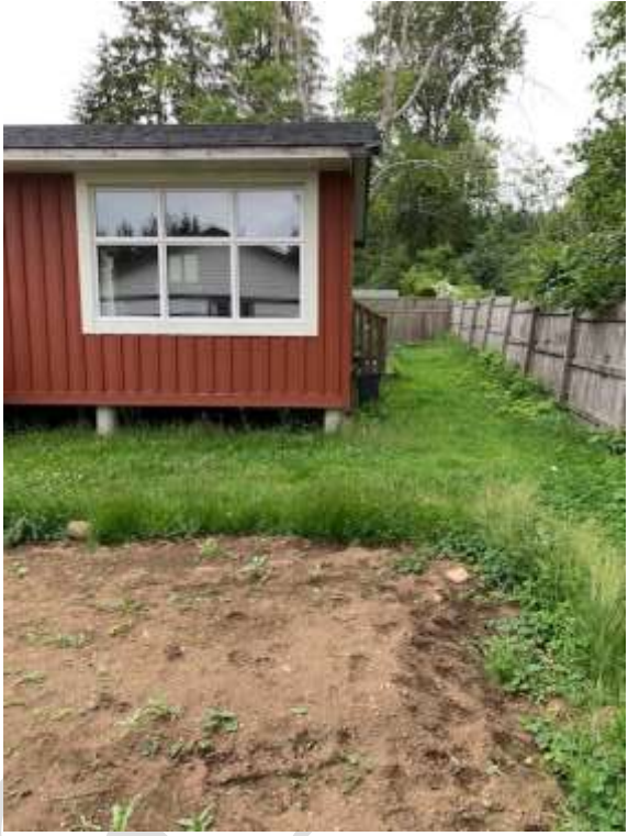
Figure 5: Accessory Building & Rear Lot Line (northern side)
